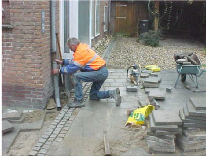
**Figure 6: de-coupling - rainwater no longer flows into the sewer system**
